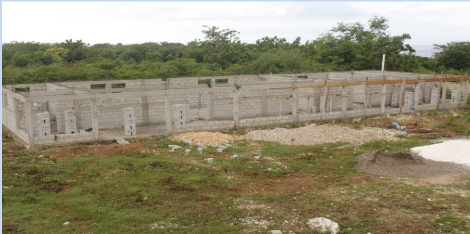
HSF Trade School Construction: As Of April 2021
