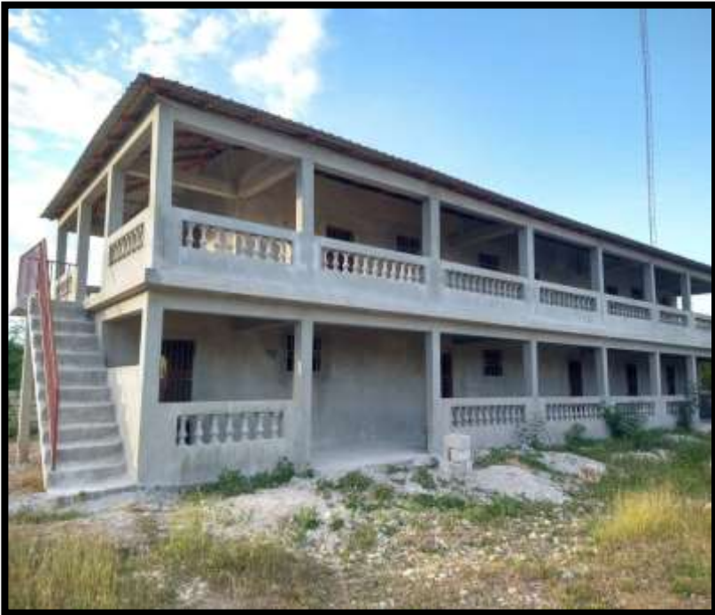
Exterior View & Stairway Leading to Second Floor
