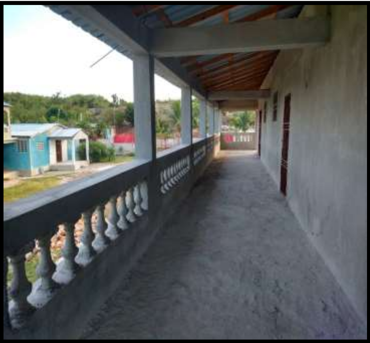
Hallway View With Steel Doors & Windows
